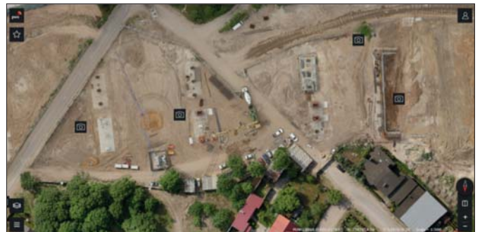
Road construction project monitoring using PwC Geospatial.App
